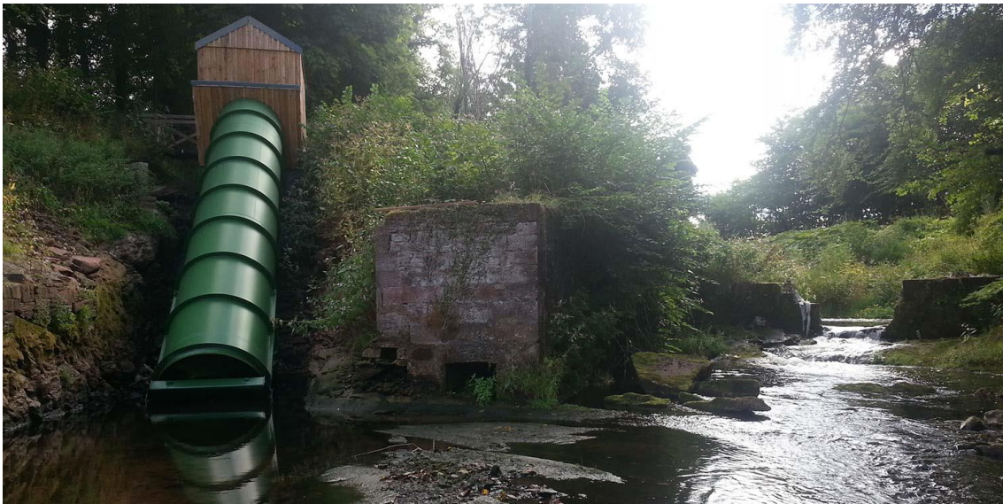
Figure 17: Photograph of 35 kW Archimedes' screw at Keithick, Perthshire, reproduced with permission (MannPower, 2015)
