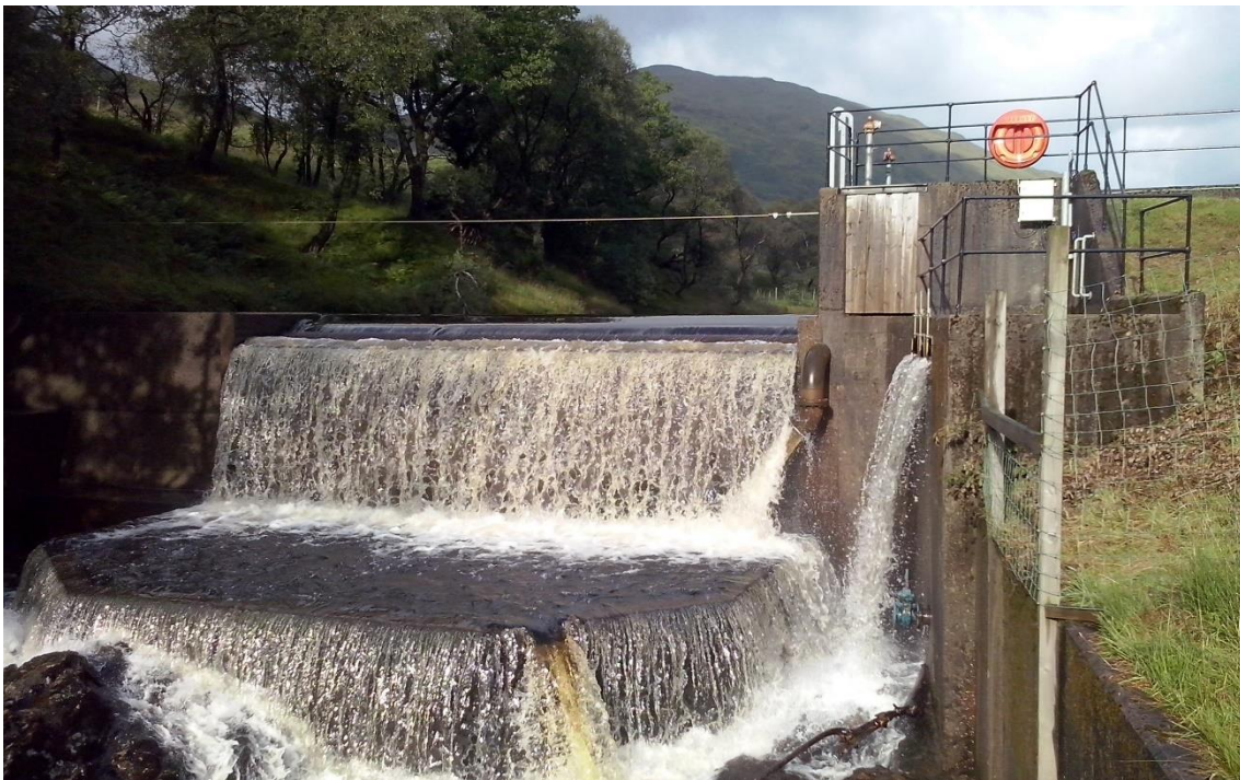
Figure 24: Author's photograph of the intake and fish pool at Inverbeg hydro scheme in Glen Douglas.
