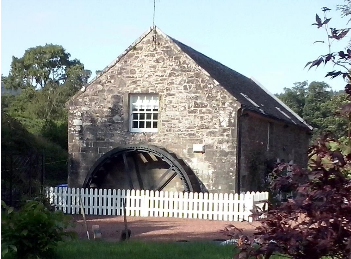
Figure 21: Author's photograph of Buchanan Mills near Drymen
