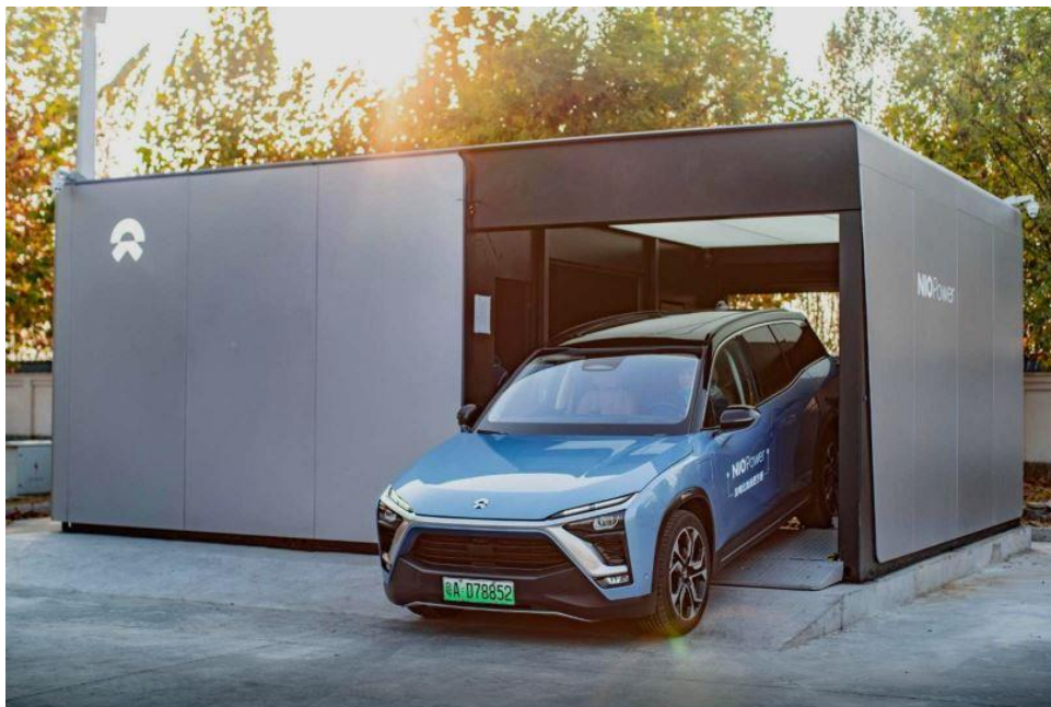
Figure 18: EV Battery Swapping Station (116)
