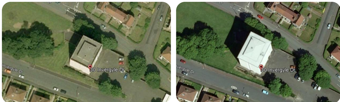
Figure 9 Satellite image from 01/01/2007 (left) and 31/05/2009 (right) (Google LLC, 2019).
