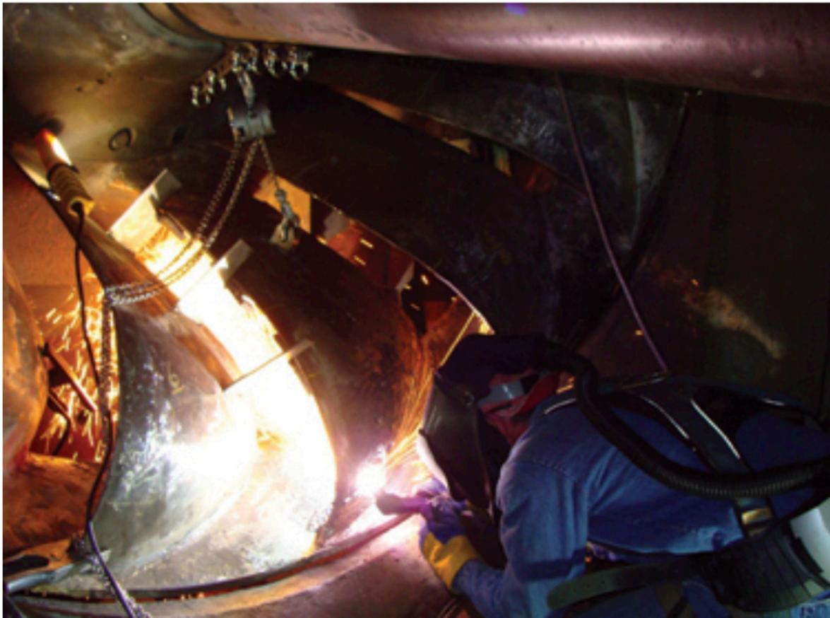
*Figure 37: Direct Removal of Francis Turbine Runner Blades (Potter, 2013)*
