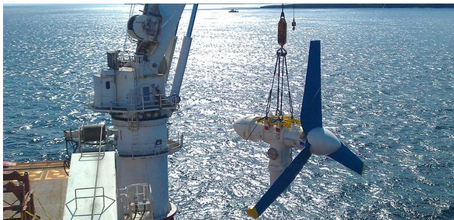
Figure 13: MeyGen Turbine being installed in the Pentland Firth (James Fisher, 2014)
