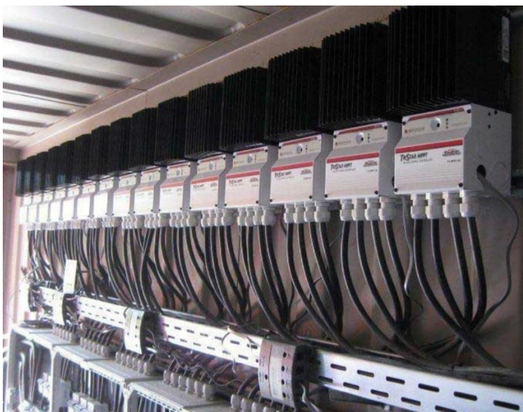
Image 3 Controllers connected in parallel [35]
