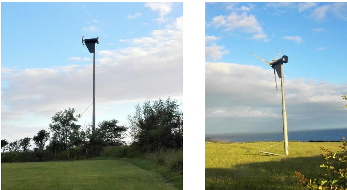
Figure 39. Wind energy systems on Arran; Small wind turbine next to Kilmory primary school (left) and turbine as a part of farm land in the south (right); pictures taken during a field trip on June 23, 2017
