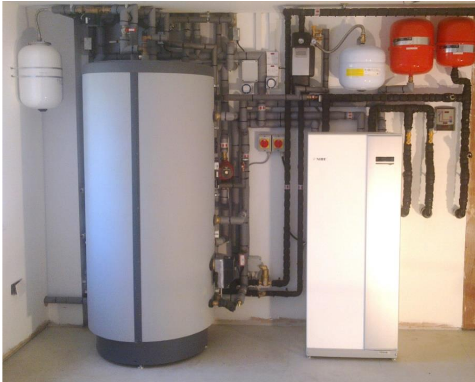
Figure 8. Hot water storage tank as a part of a conventional heat pump system ( Solo Heating Installations, 2017 )
