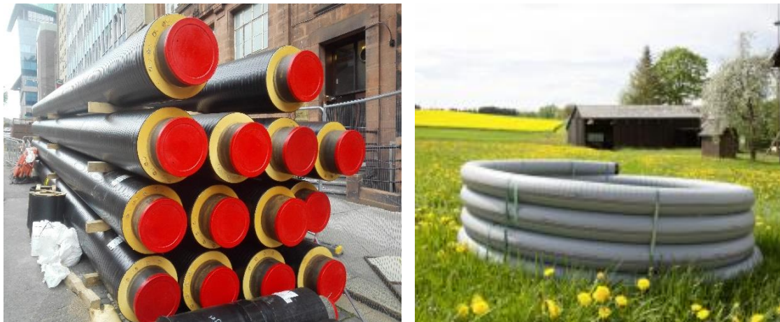
Figure 51. Steel pipes with a large diameter used for district heating scheme at the University of Strathclyde (left) and bonded pipes with PU foam (right) (Rehau, 2017)
