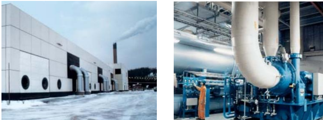
Figure 13. The largest water source heat pump scheme in the world - 180MW capacity operating in Stockholm, Sweden ( Friothersm, 2015 )
