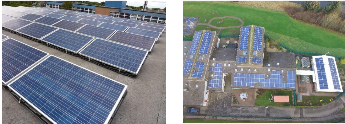
Figure 26. Solar PV installations as a part of ECSC scheme; Davidson mains primary school 35 kW (left) and Ratho primary school 80 kW (right) (ECSC, 2017)
