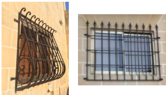
Figure 2.4. Steel bars limiting entrance through the windows. Source: Author
