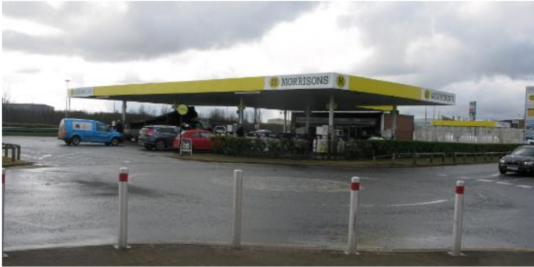
Figure 3.2.3: Morrison shopping and petrol station
