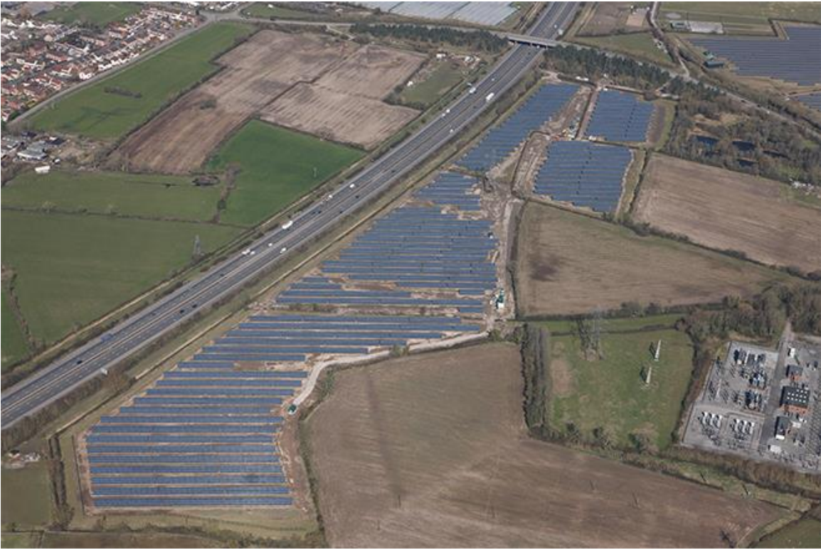
Figure 2.4: the top-view Park Wall 5 MW Solar Farm
