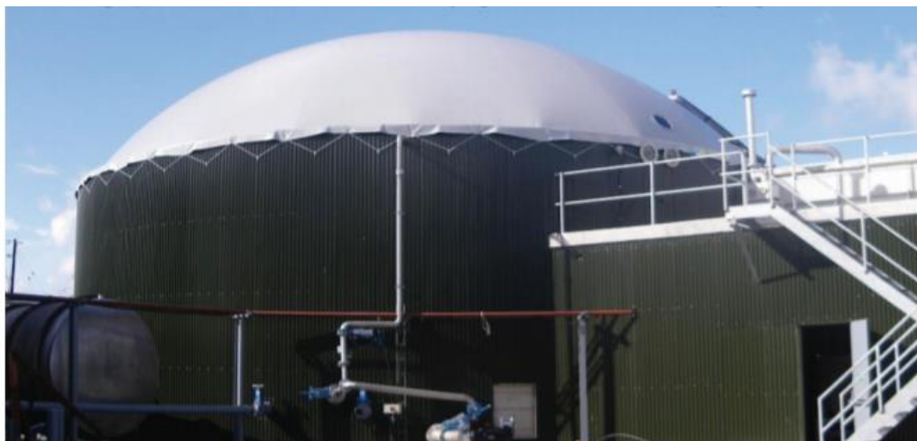
Figure 6.5. Primary digester (source: Biogas plant McDonnell Farms Limited)
