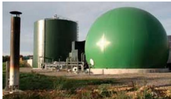
Figure 2.2. 1480m 3 AD plant on a UK farm processing slurry, maize and glycerol (Source: Community by Design)
