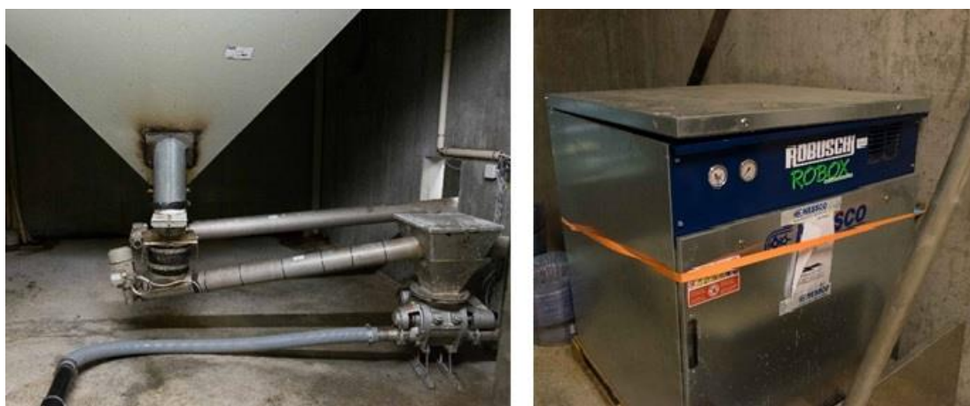
Figure 28 Feeding system at Teistholmen salmon farm. Left: Bottom of the feed silo and the progressive cavity pump. Right: compressor unit, driving the feeding system.
