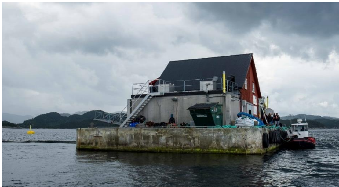
Figure 25 The feed barge at Teistholmen Salmon farm, where the feeding system, crane, monitoring station and kitchen is kept. The electrical demand profile created is based on this salmon farm.
