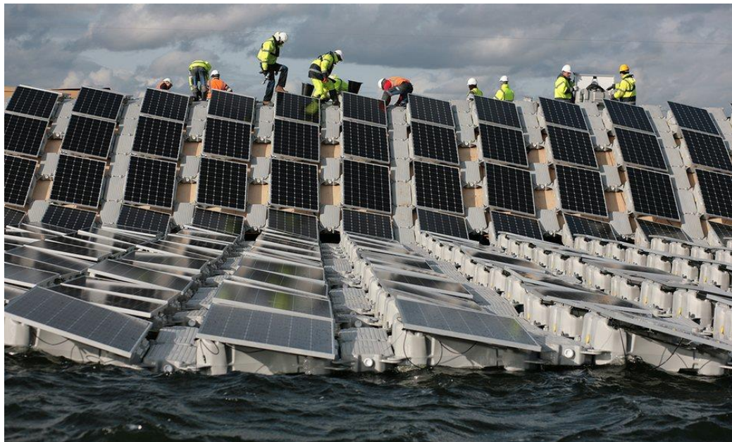
Figure 17 PV panels on floating modules on the Queen Elizabeth II reservoir outside London. This is a possible solution for salmon farms (Godwin, 2016).
