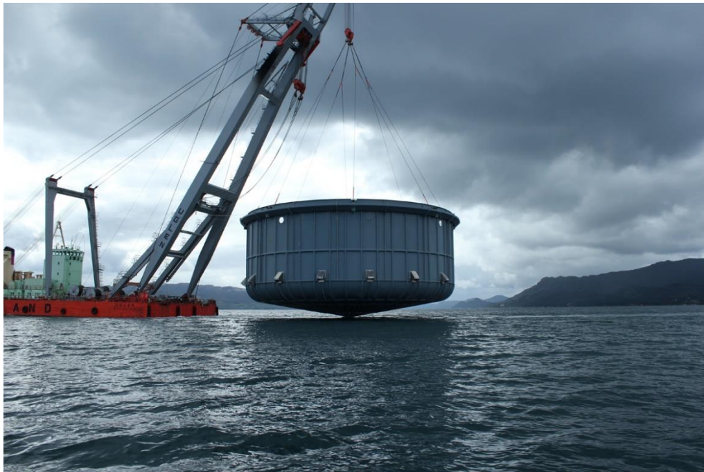
Figure 10 Closed cage ocean farm in Norway. No openings, so this would operate like a closed system with pumps circulating the water (Marine Harvest, 2013).
