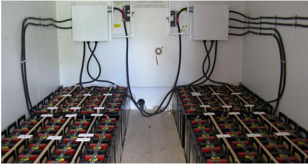
Figure 22 A battery bank is an example of a storage option. In this picture, Lead-Acid batteries are used to store the electricity of a renewable energy system (Schauberger, 2015).
