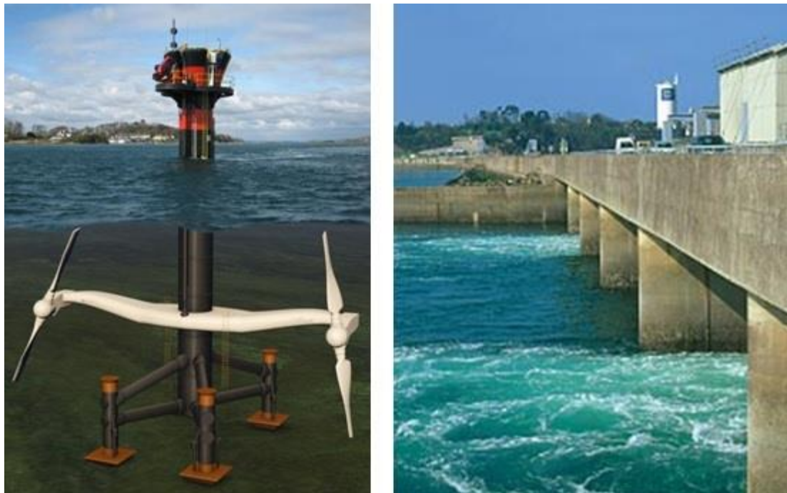
Figure 20 Two different concepts for harvesting tidal energy. To the left is a 1.2MW Sea Gen tidal stream generator (Sea Gen, 2013). To the right is the 240 MW Rance tidal power station in France (REUK, 1998)
