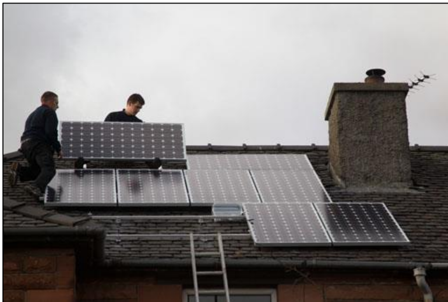
Figure 14 Installing rooftop PV panels (Photoscot, 2013)
