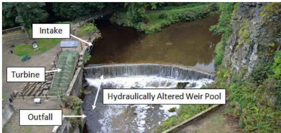
Figure 18 Low-head run-of-river hydropower scheme (Anderson et al., 2014)
