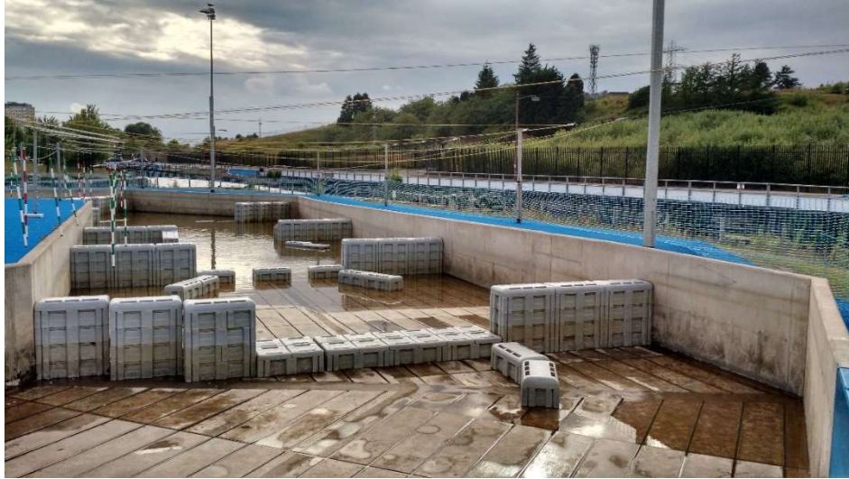
Figure 6 Modular blocks can be used to modify the flow of water down the course
