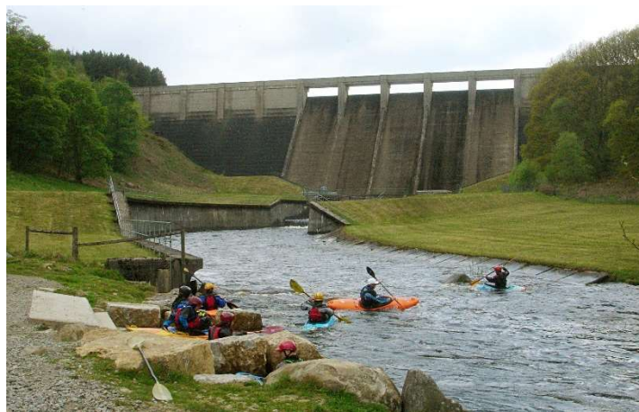
Figure 7 River Washburn below Thruscross Reservoir Dam
