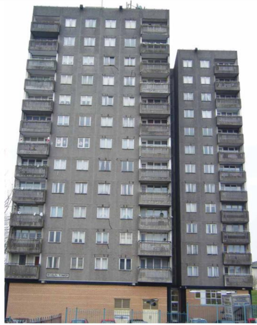
Figure 2: Tower block before refurbishment (D&B Facades, 2013)
