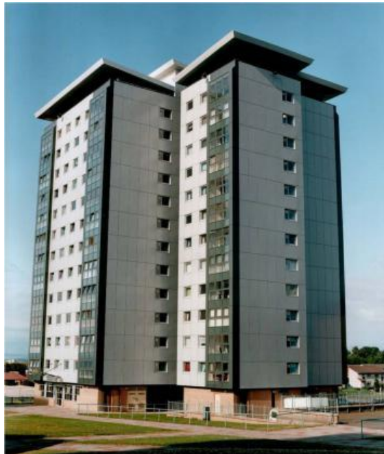
Figure 3: Tower block post refurbishment (RIAS, 2016)
