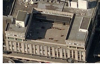
(b) Southern façade
