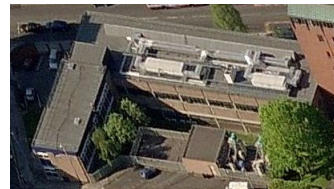
(b) Southern façade
