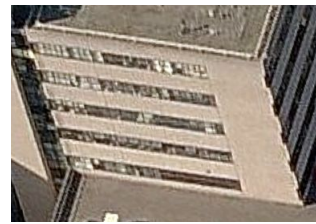
(b) Southern façade
