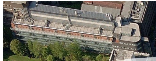
(b) Southern façade
