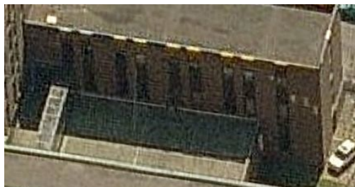
(a) Northern façade
