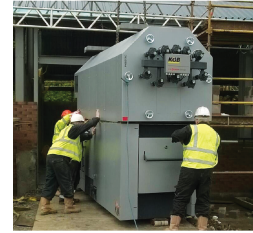
(b) The 740kW biomass boiler being installed for district heating
