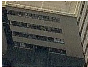
(a) Northern façade
