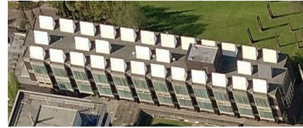
(b) Southern façade
