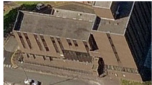
(b) Southern façade
