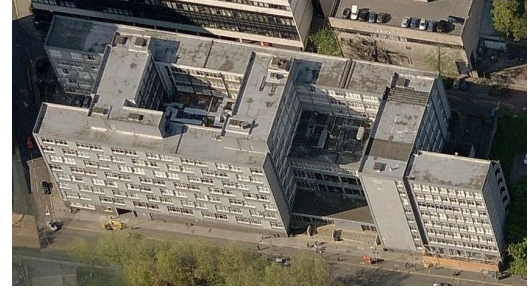
(b) Southern façade
