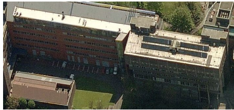
(a) Northern façade
