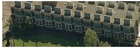
(a) Northern façade
