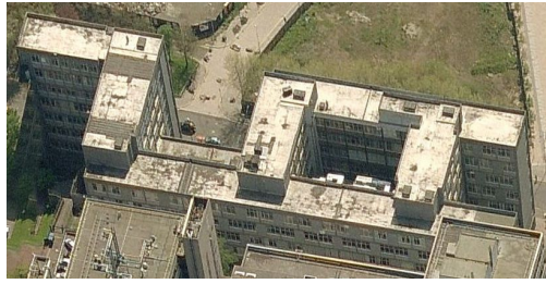
(a) Northern façade
