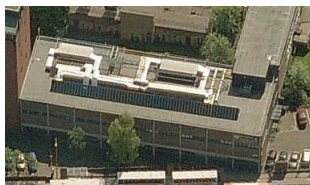
(a) Northern façade
