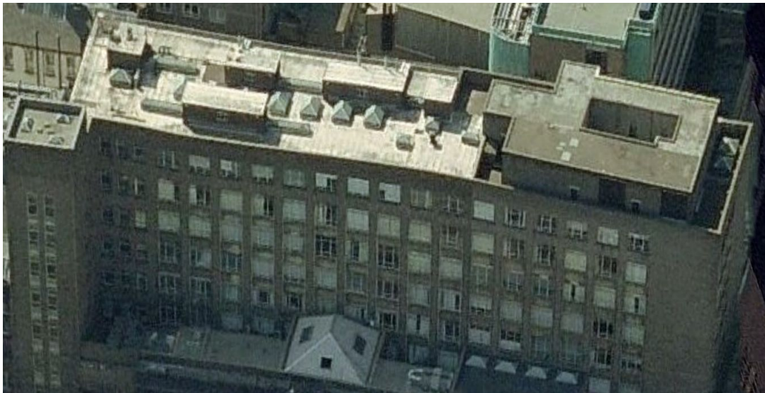
Figure 20: Aerial image of the eastern façade of the James Weir Building
