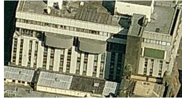
(c) Western façade
