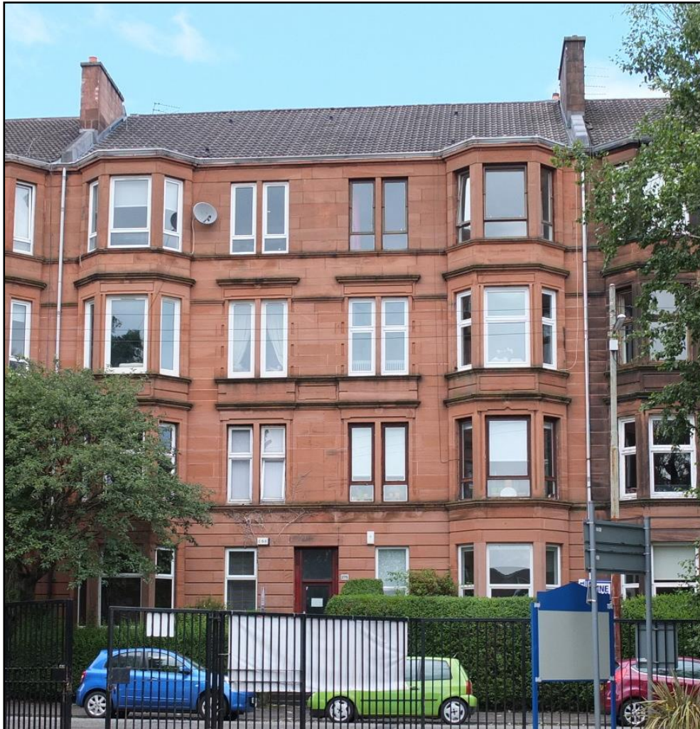
Figure 15 Photo of typical Glasgow tenement housing, for “Onslow” scenario
