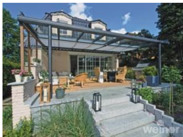
Figure 16: An example of an external glazed canopy (The garage door, 2016).
