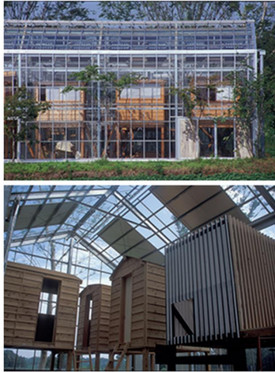
Figure 43: Millennium City - wooden cabins in greenhouse (Fifthworld-inc.com)
