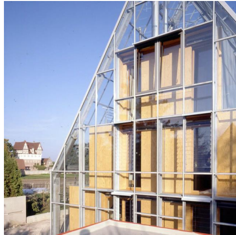
Figure 47: Gable with specially developed window constructions (Niederwöhrmeier + Kief Freie Architekten BDA und Stadtplaner)
