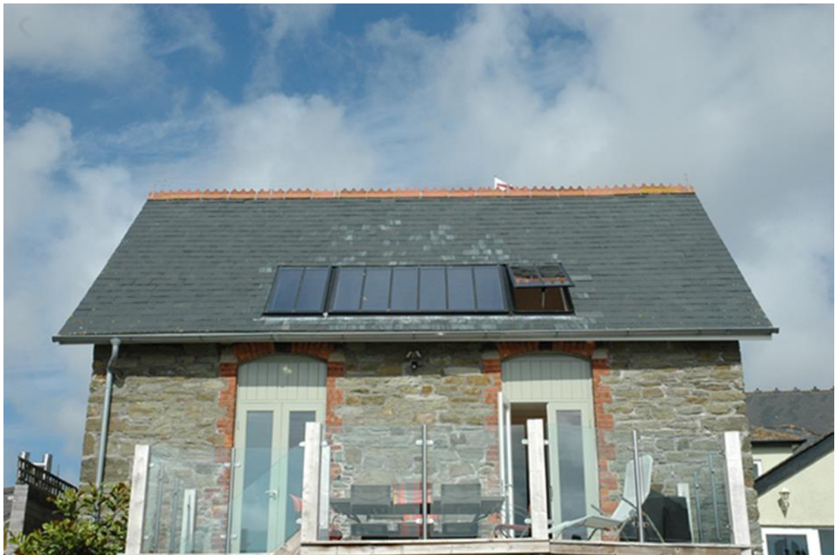
Figure 17: An example of a typical skylight (lumenrooflight, 2016).
