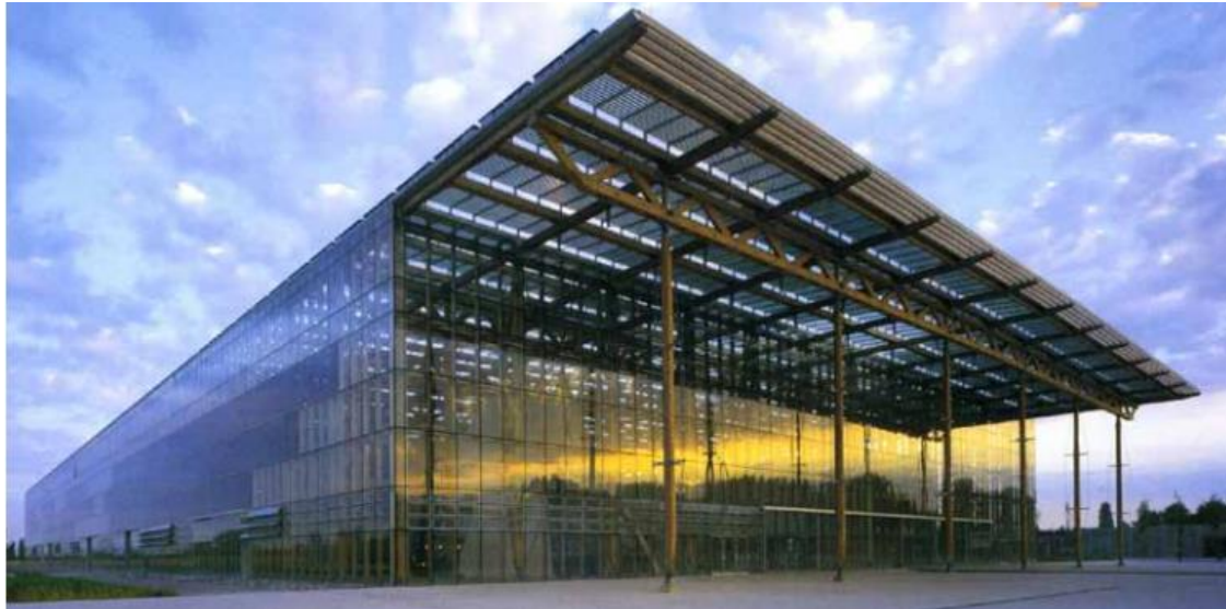
Figure 48: View of the Academy Mont-Cenis building in Herne (Academy Mont-Cenis Herne)
