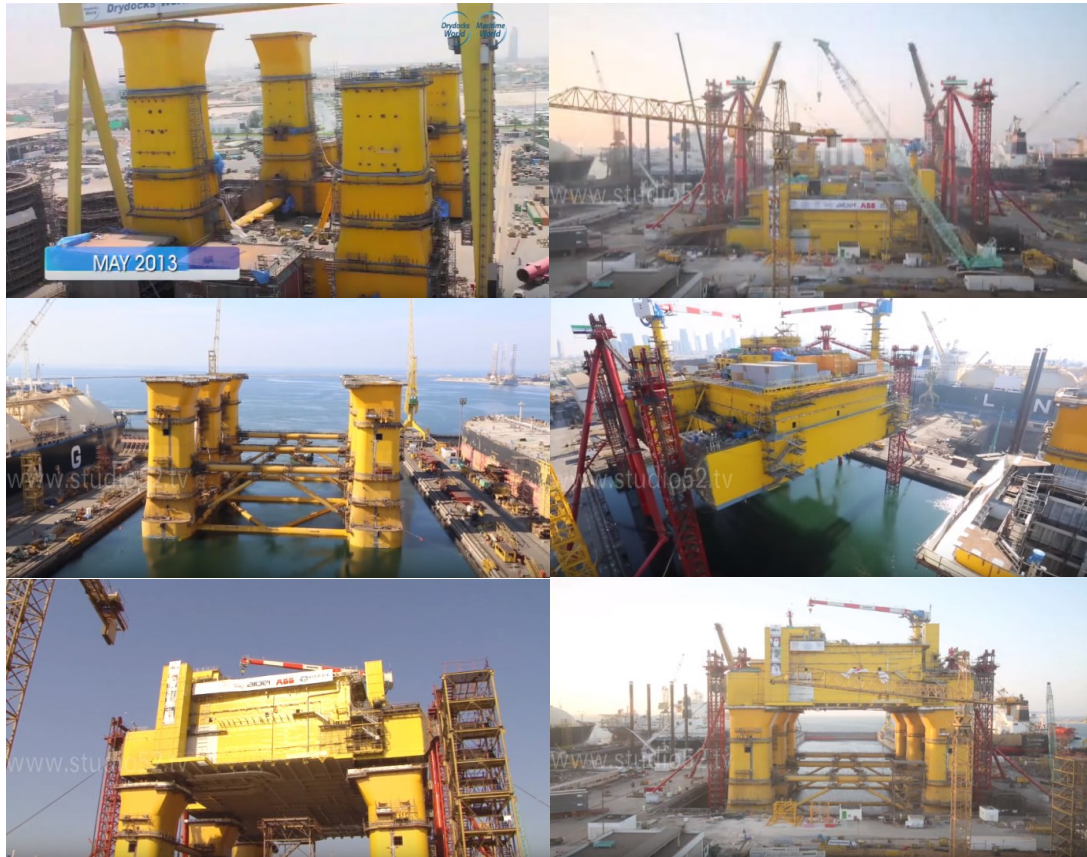
Figure 24: Dolwin Beta Fabrication Sequence (28)
