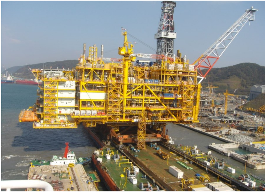
Figure 5: Topside is skidded onto the HYSY229 launch barge (8)
