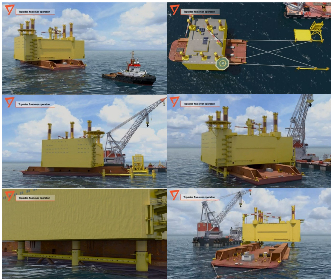
Figure 3: Sylwin Alpha, float-over installation sequence (6)
