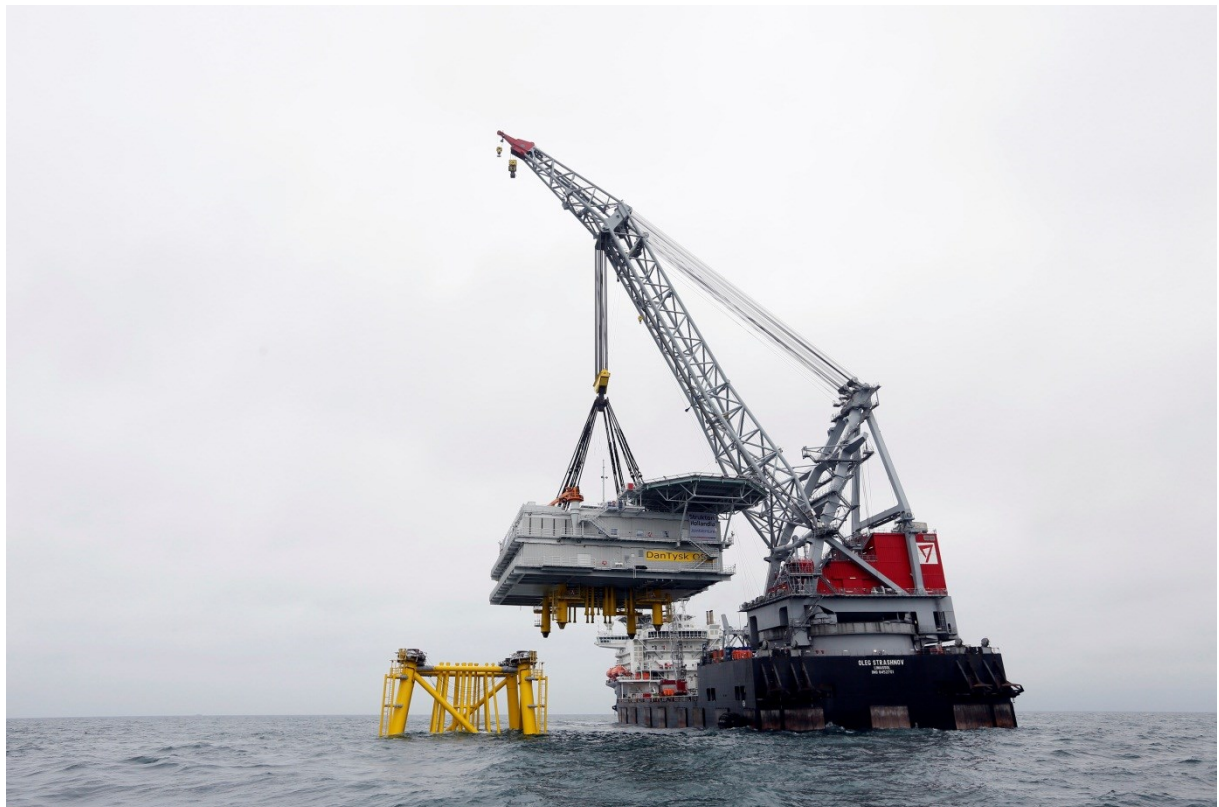
Figure 9: Dantysk OSS lifting operation by SHL (11)
