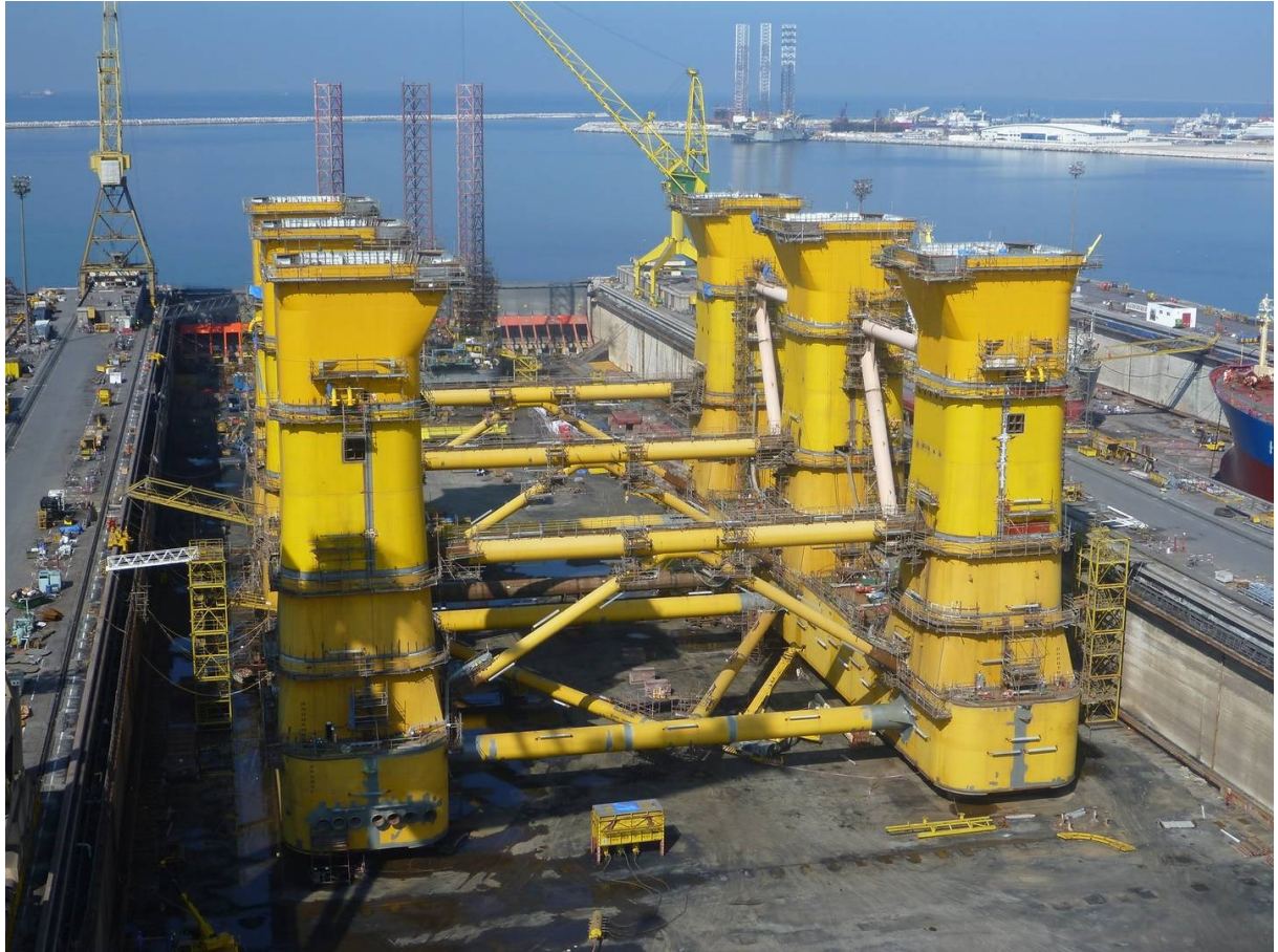
Figure 23: Fabrication of Dolwin beta bracings, columns and pontoons on drydock (27)
