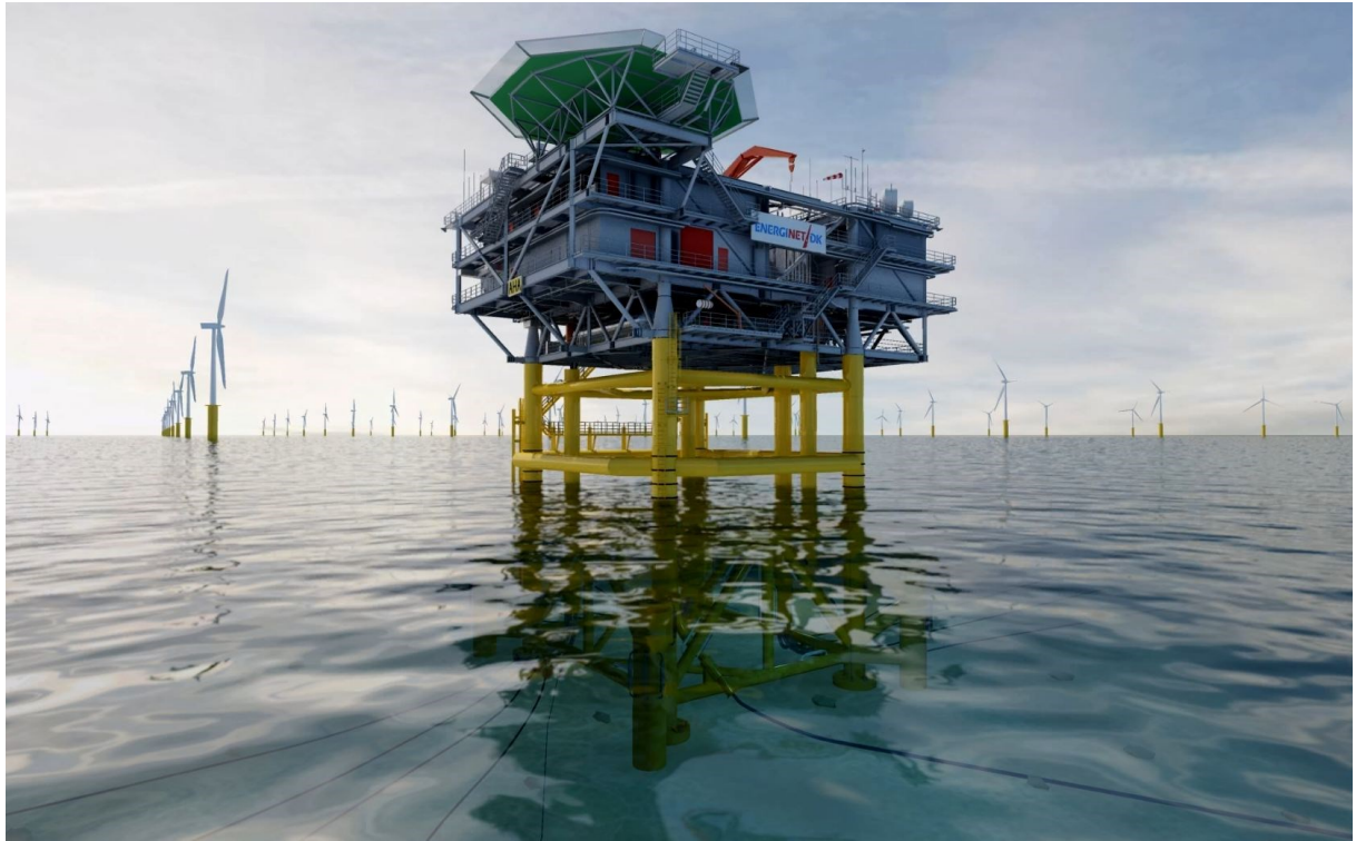
Figure 2: Anholt Offshore Substation (4)
