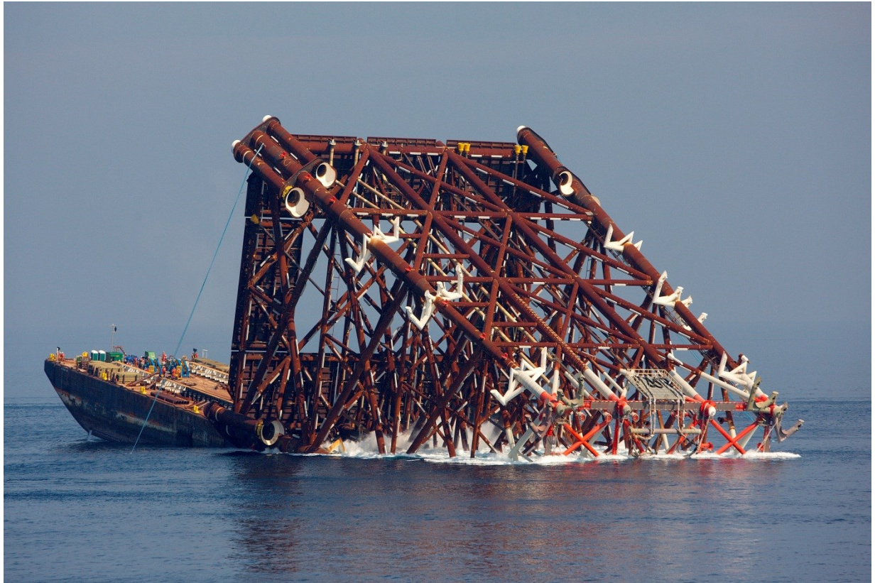
Figure 12: Launching Operation. North Field Alpha Project (Qatar) (15)
