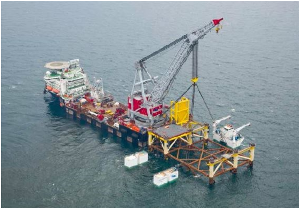
Figure 11: Lift float, Sylwin Alpha Jacket Installation (14)
