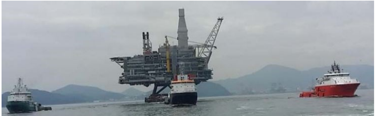
Figure 6 Oil and Gas Float-over Topside transported on a Heerema Barge (9)
