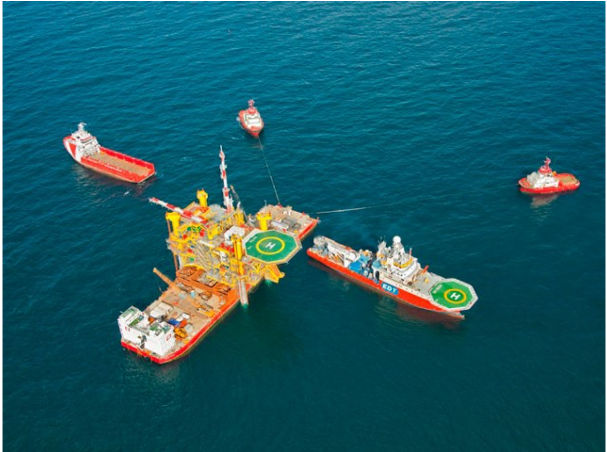
Figure 16: F3-FA Installation, SEU assisted by barge (19)
