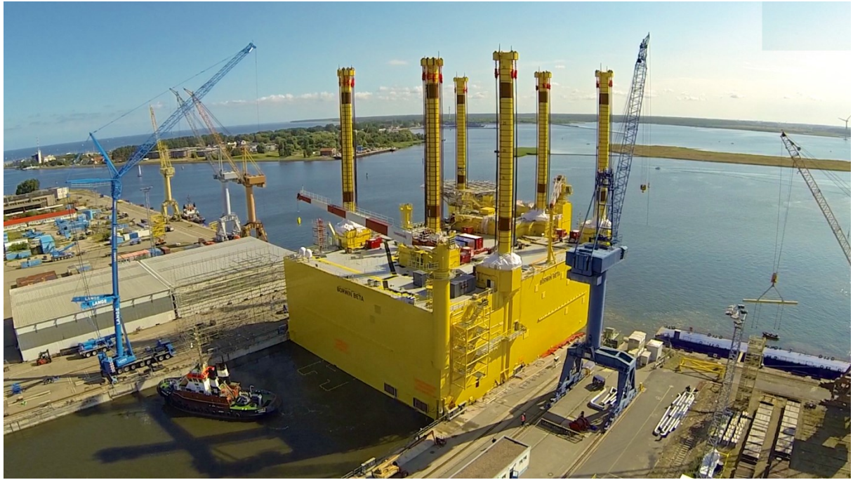
Figure 19: Borwin Beta OSS assisted by tug vessel inside dry-dock (21)
