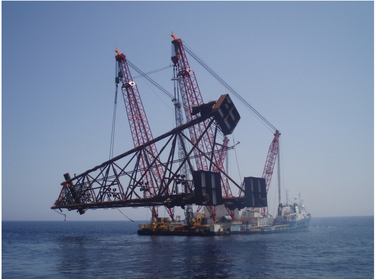
Figure 10: Double Hook Lifting Operation by Rambiz HVL (12)
