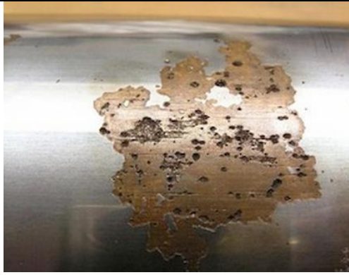
Figure 9 Pitting Corrosion Example 1
