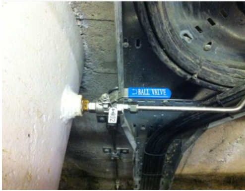
Figure 4 Galvanic Corrosion - Example 1
