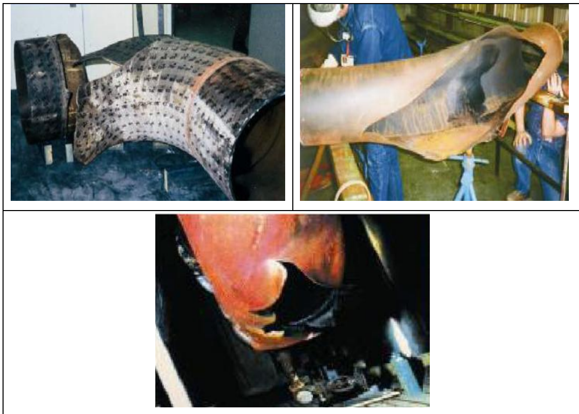
Figure 16 Examples of Flow Assisted Corrosion - (Ahmed, 2010)
