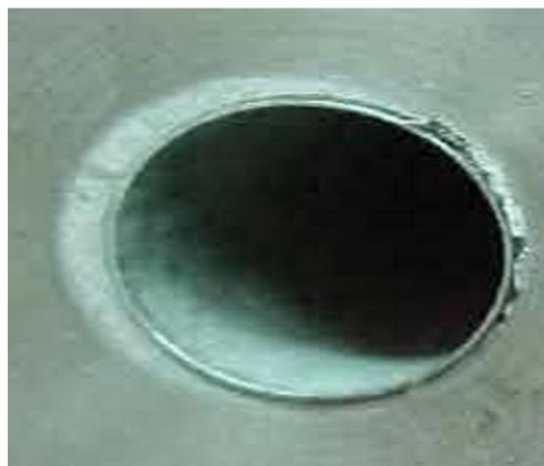
Figure 6 Crevice Corrosion Example 1
