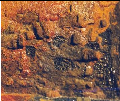
Figure 11 Pitting Corrosion Example 3
