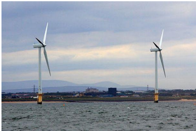
Figure 11 - Britain's First Offshore Wind Farm at Blyth (Black, 2009)
