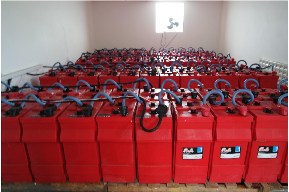
Figure 15 - The Battery Configuration on Eigg
