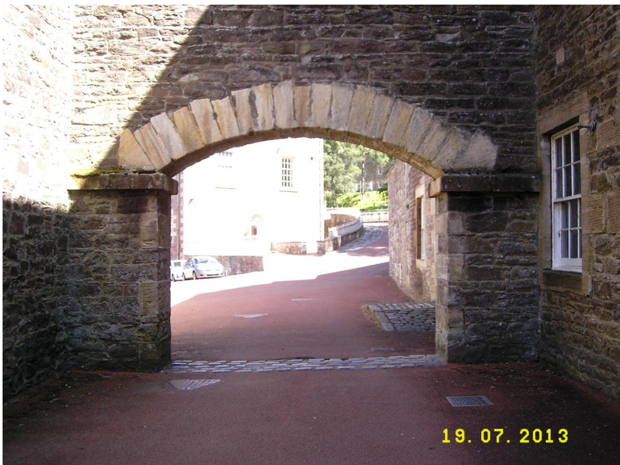
Fig 18 One of the retaining arches impeding access to larger vehicles.
