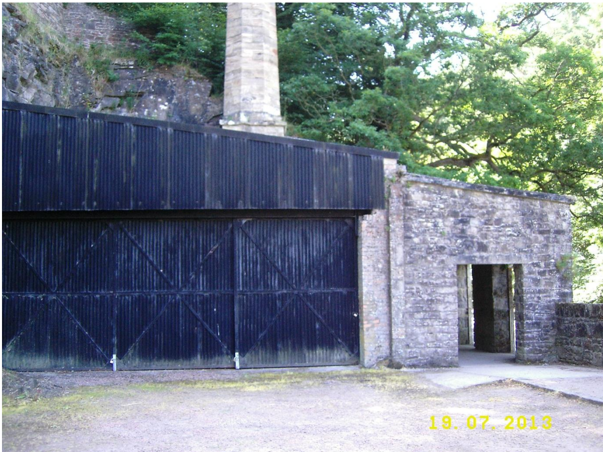
Fig 17 The Proposed Location for the Biomass Boiler System.
