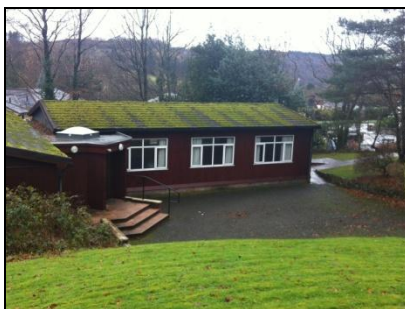
Strathblane Church Rooms, Pop: 1,964.
