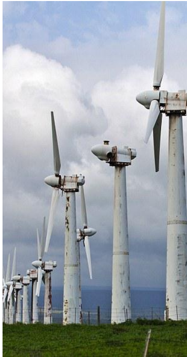
Figure 9- Rusted turbines
