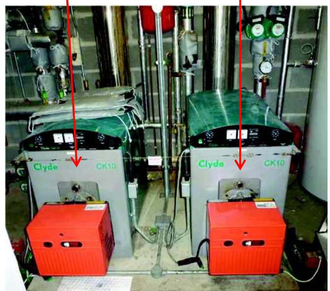
Figure 6-3: Oil Boilers
