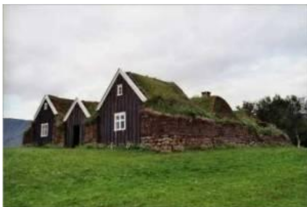
Figure 11: Icelandic house with passive heating technology (Passipedia, 2013)
