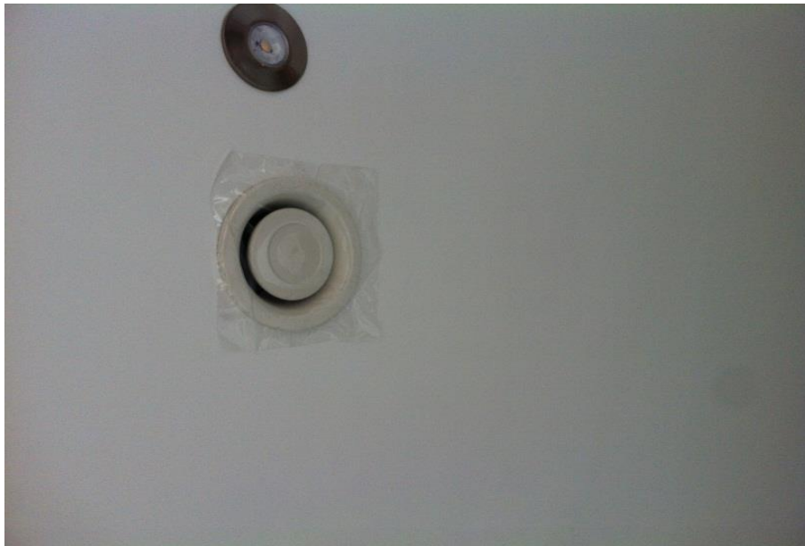
Figure 4.5 – Picture of a sealed fan point
