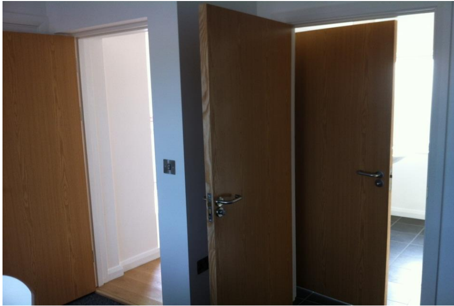
Figure 4.6 – Picture of internal doors in the house open
