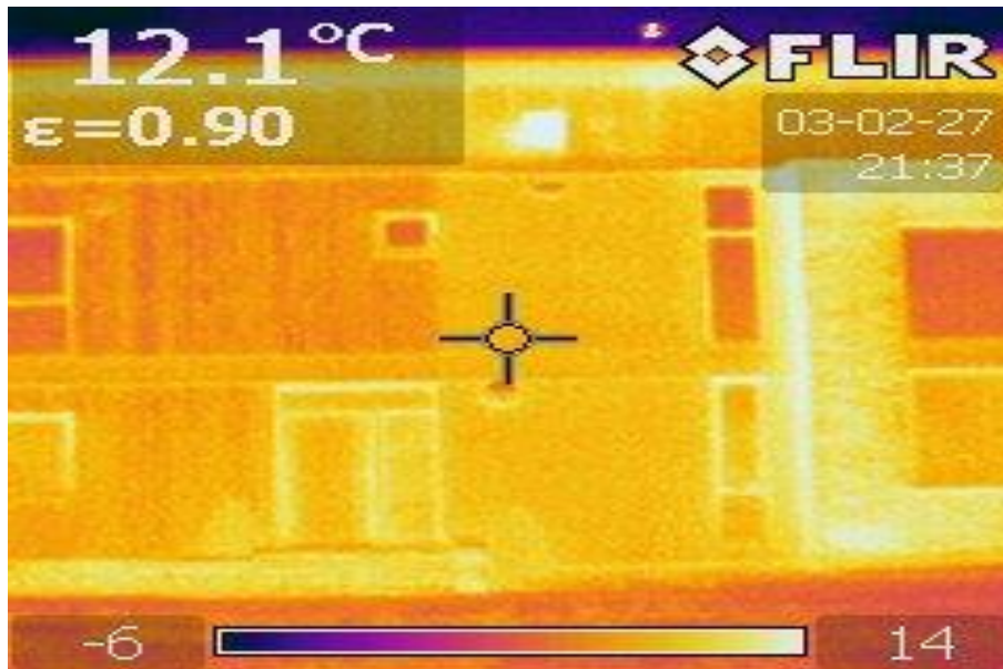
Figure 4.13 – Thermographic image of north facing wall
