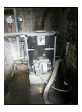
Gas heaters are used occasionally when double casting. (2 units simultaneously cast, twice per day) and are also used during winter. There are two gas heaters with a thermal output of 82.43 kW and 102.3 kW. However, the amount of fuel used varies depending on the number of precast units required and the ambient temperature.
