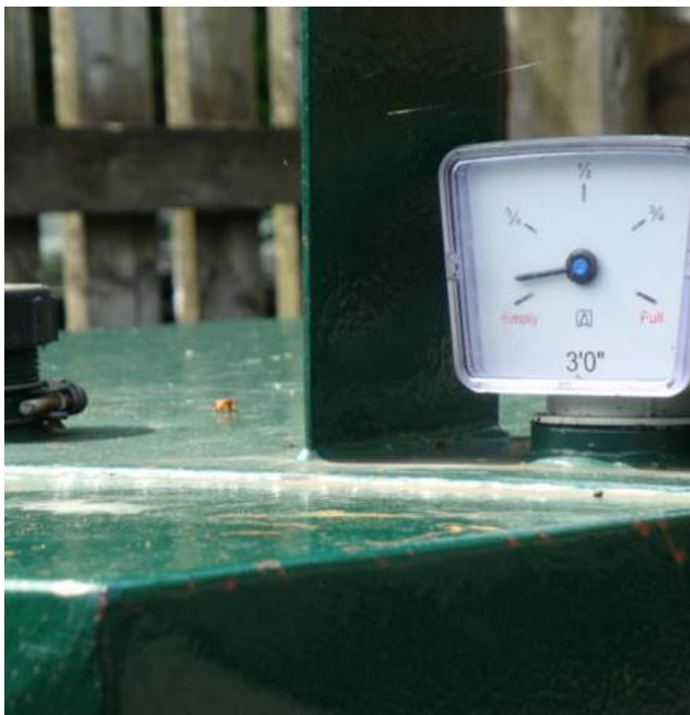
Figure 6-7 Oil tank gauges in situ, illustrating access challenges
