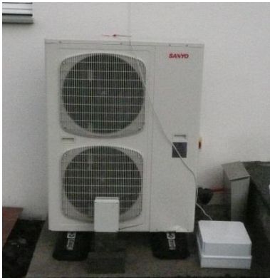
fig. 47- The Sanyo CO 2 heat pump in Oban
