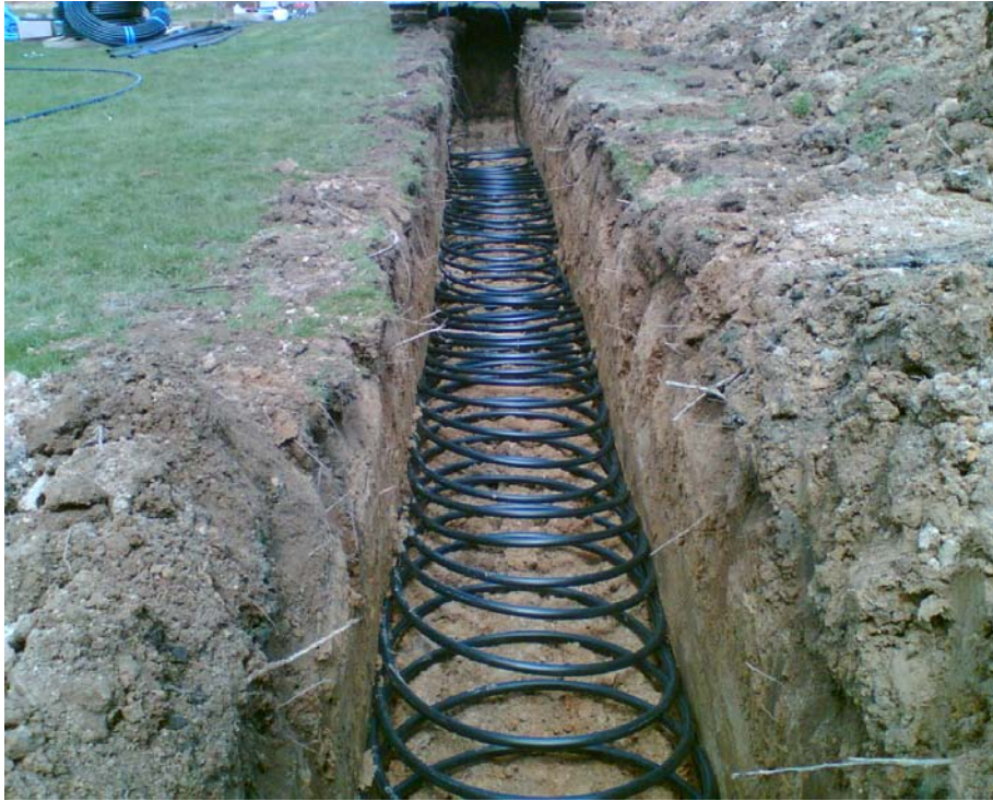
Figure 14 - Ground Source Slinky Closed Loop [33]
