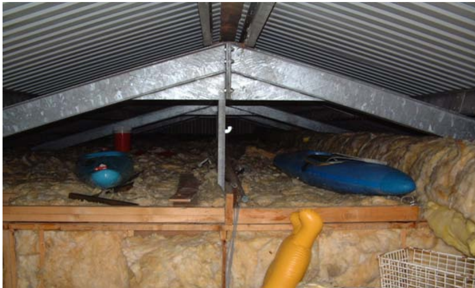
Figure 31 - Swimming Pool Roof Space
