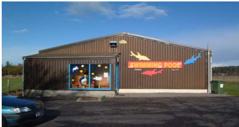
Figure 28 - Poolewe Swimming Pool Front Entrance
