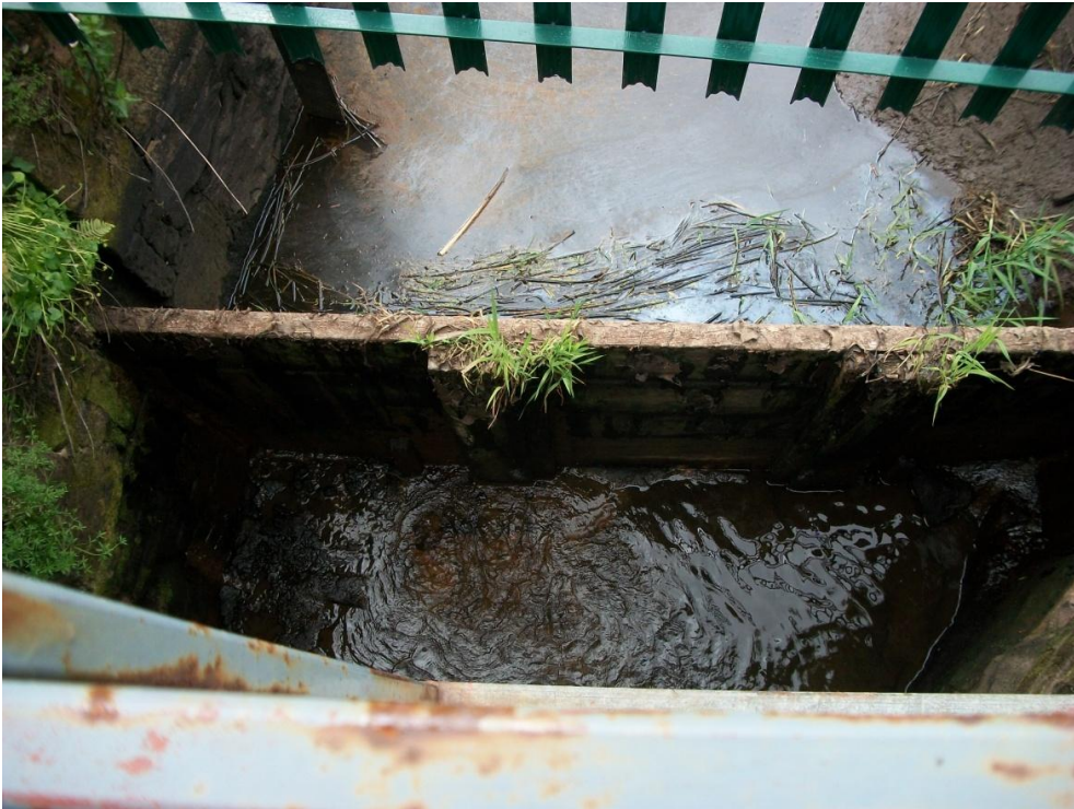
B-1: View of small wooden dam next to embankment
