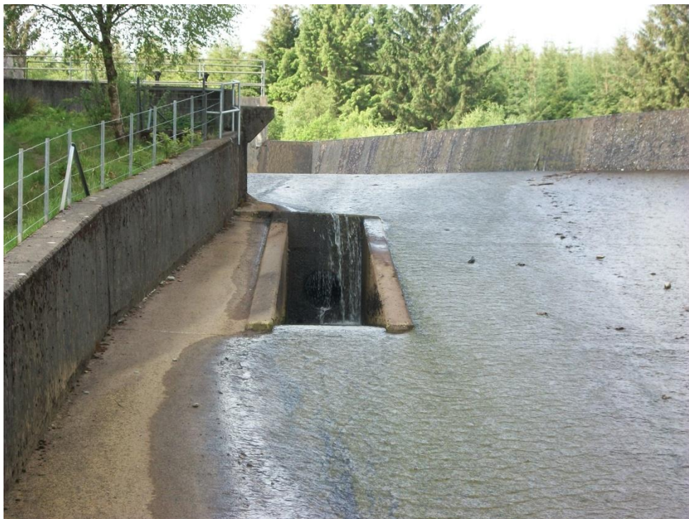
A-2: View of chute and scour valve exit
