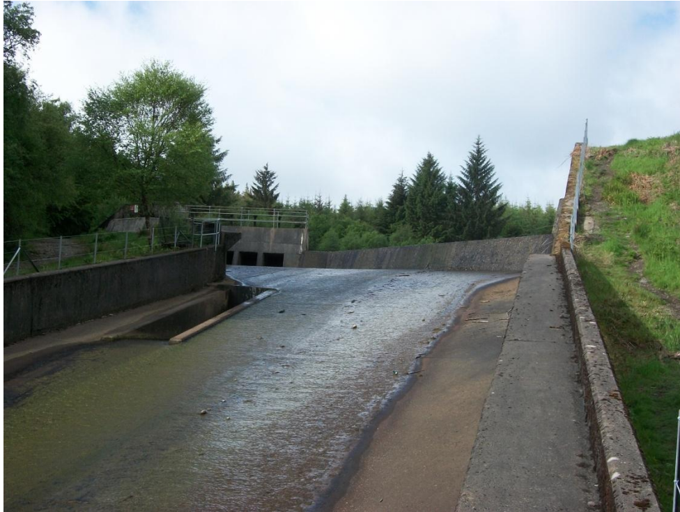
A-1: View of weir and chute from footbridge
