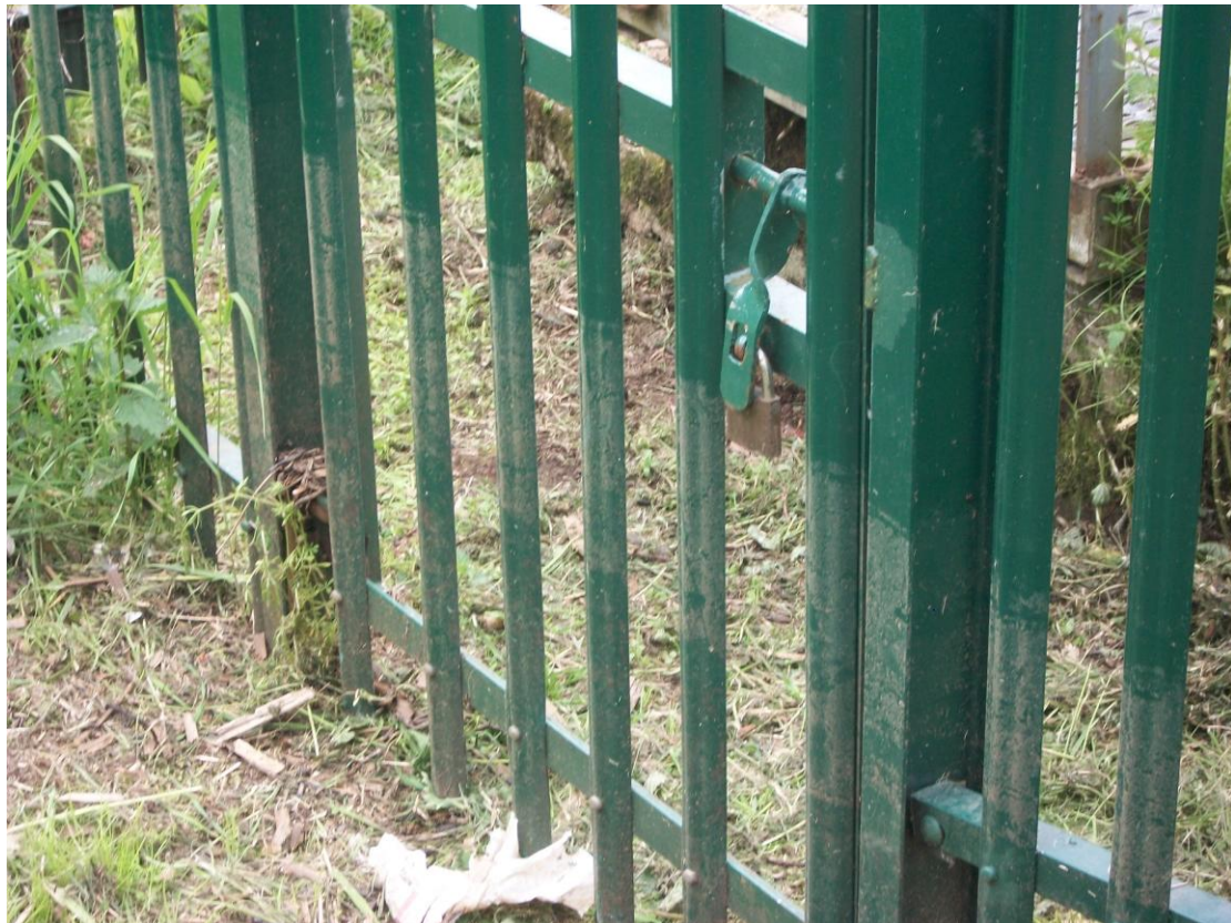
Figure 36: High water mark left after recent flooding
