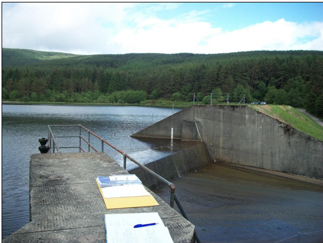
Figure 27: Earth embankment dam (background) concrete weir (foreground)
