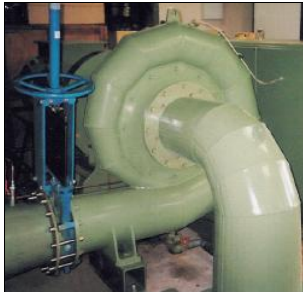
Figure 18: Horizontal axis Francis turbine (11)
