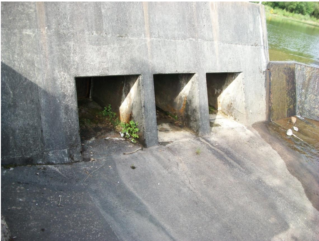
A-6: Close up of overflow sluice gates
