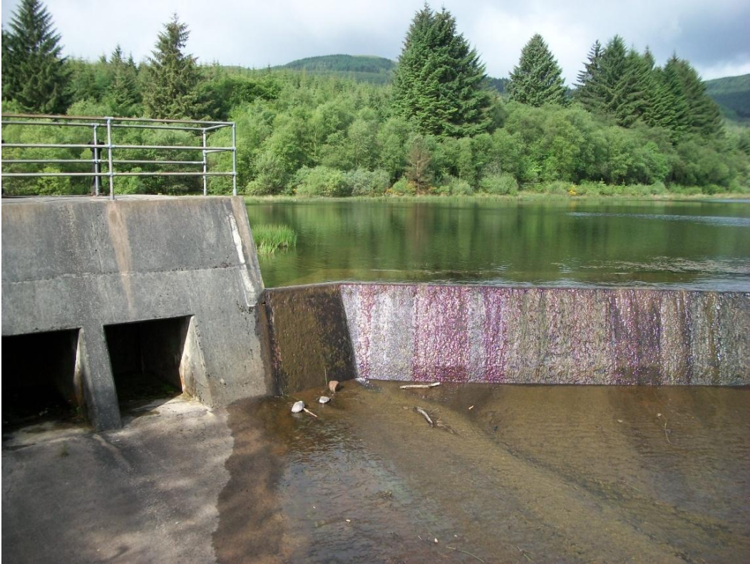
A-5: View of spillway and overflow sluice gates
