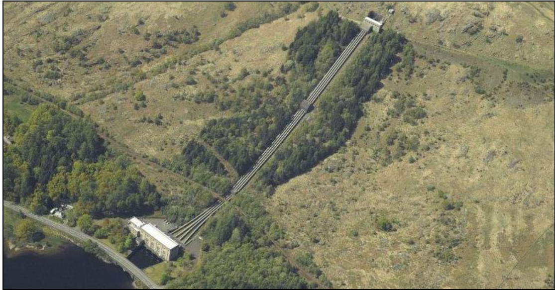
Figure 8: Loch Sloy power station (7)
