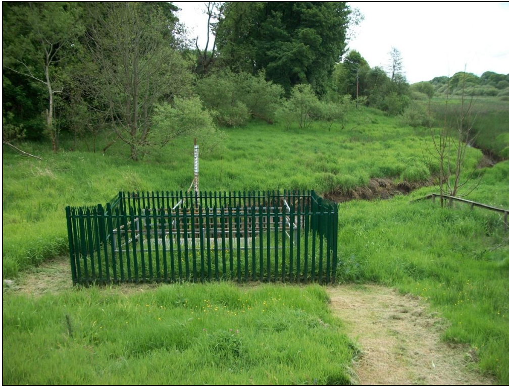
Figure 34: View of water course entering the earth embankment dam
