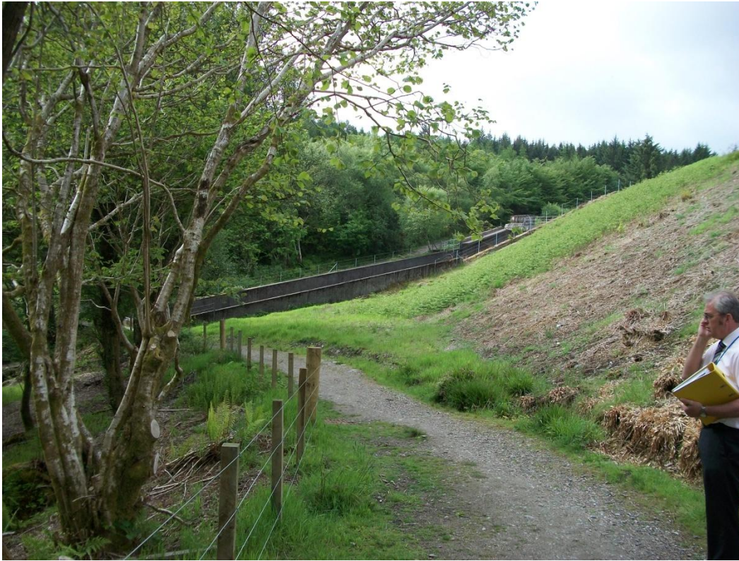
A-9: Earth embankment and concrete chute
