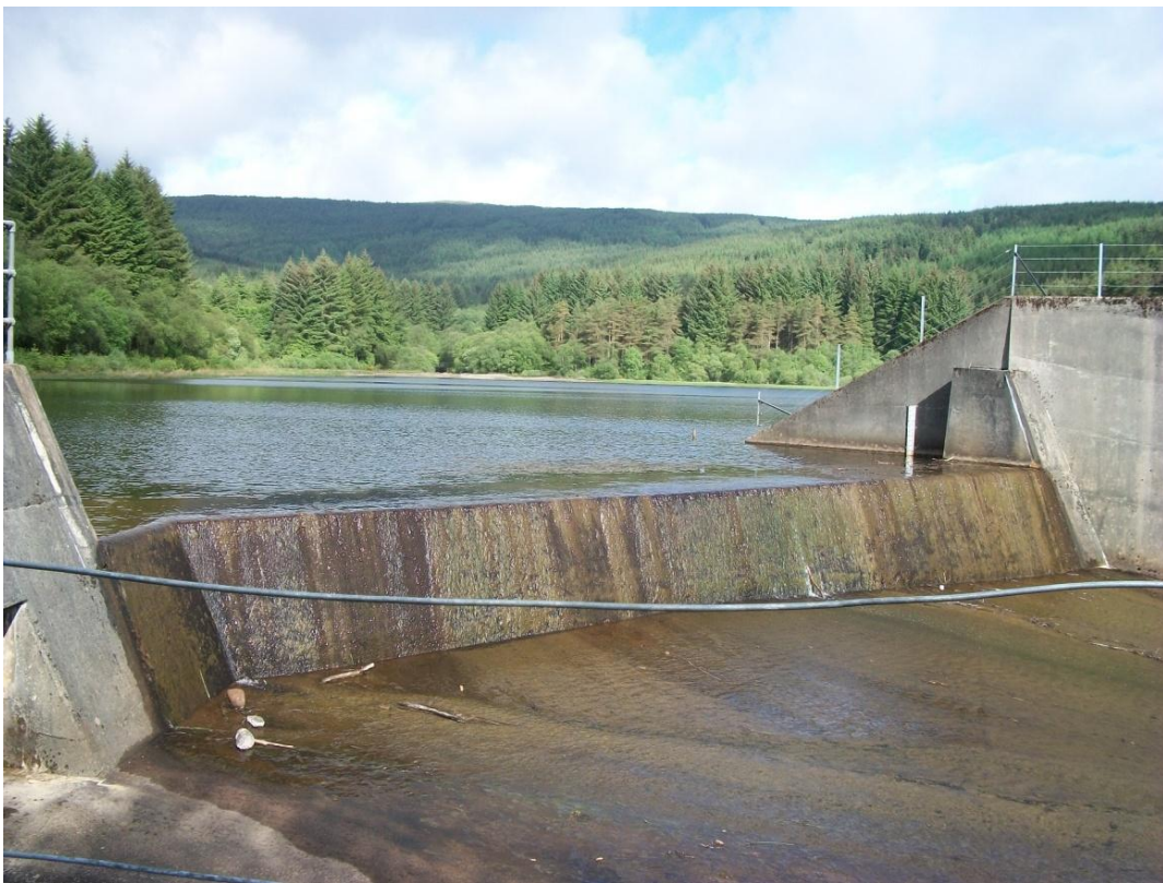
A-4: View of main weir spillway
