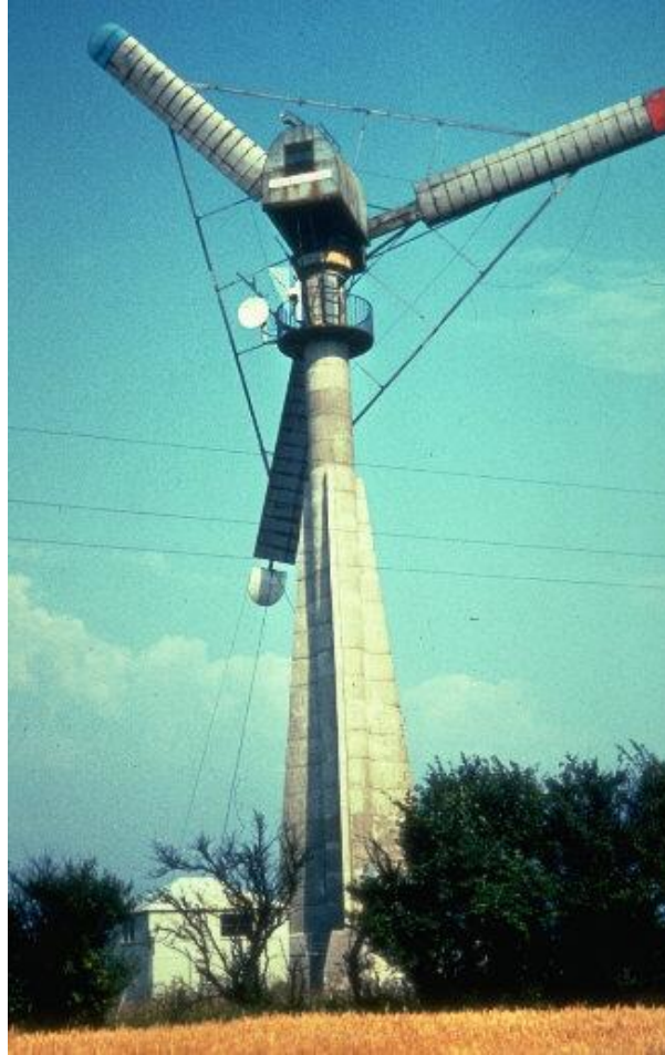
Figure 4: 200 kW Gedser Mill wind turbine, Denmark
