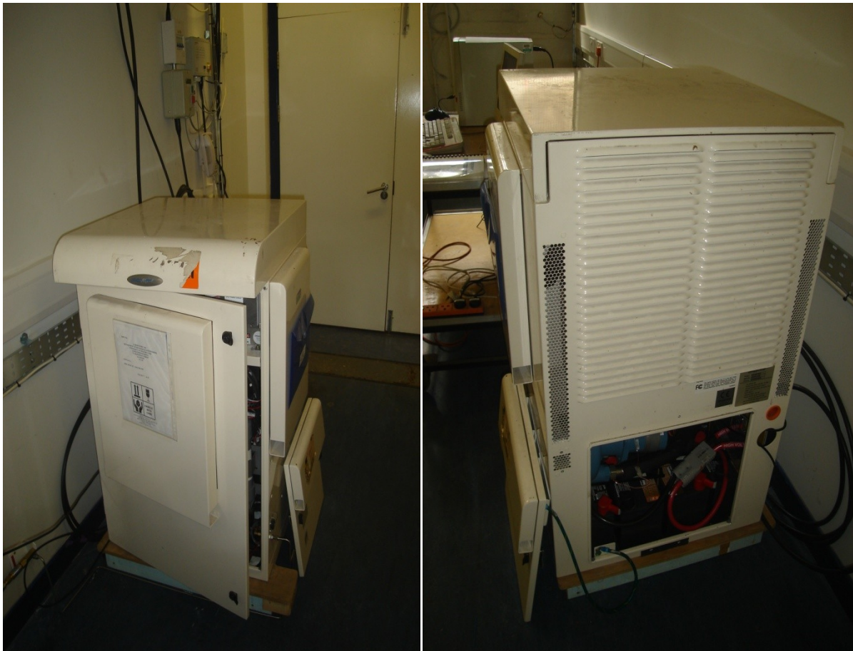
Figure 5.1.a the GenCore® 5B48 Fuel Cell System
