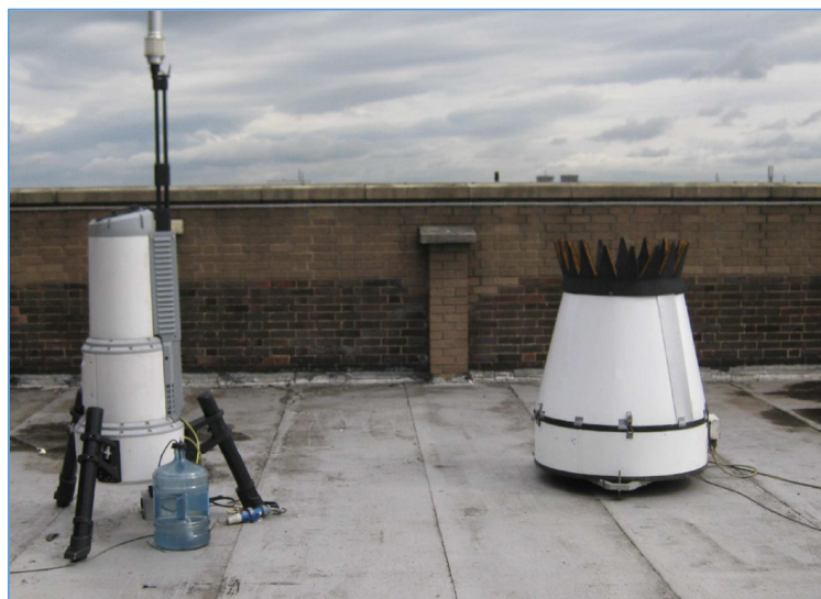
Figure 24 - Siting on the roof
