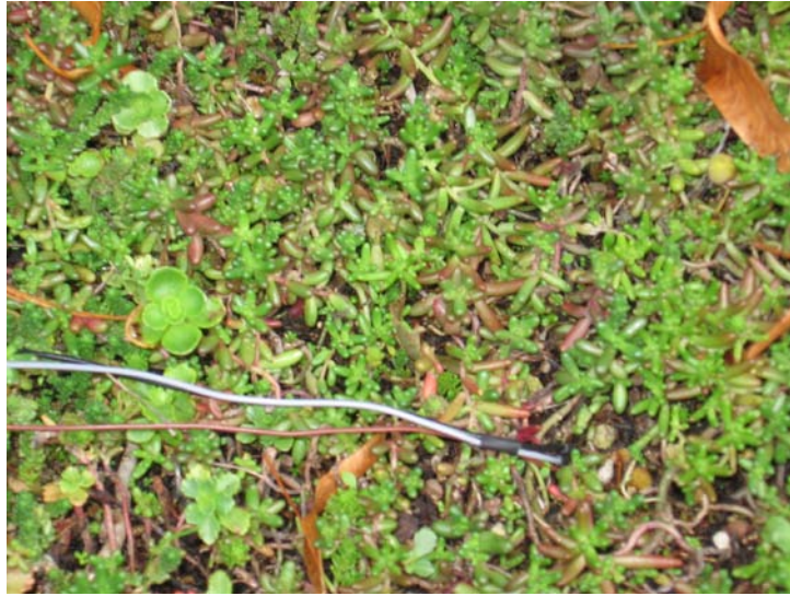
Figure 32: Humidity Sensor Located in Substrate
