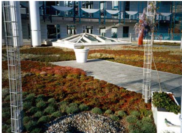
Figure 4: Semi-Intensive Green Roof (Merano, Italy) [5]
