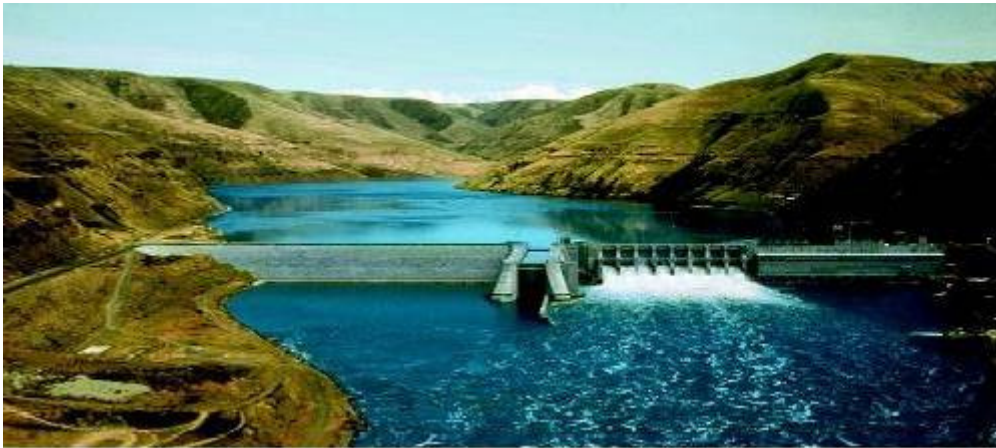
Fig. 4.2: Run-of-the-river scheme: The Lower Granite Dam, Washington. (Source: [25])
