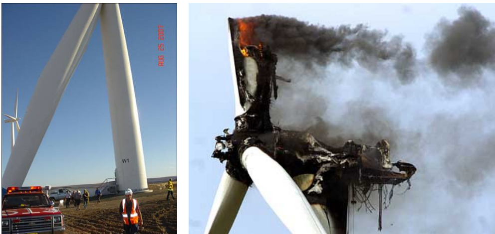
Fig. 3.8: Collapsed wind turbine tower (left) and turbine fire (right) (Source: [23], [24])
