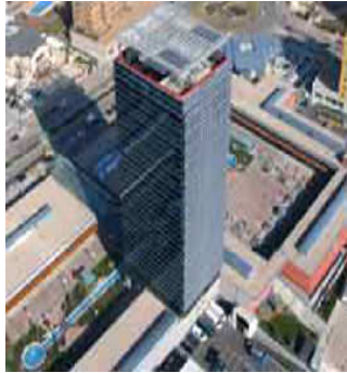
Photo 1 PV installation in Torre, Garena/ Spain
