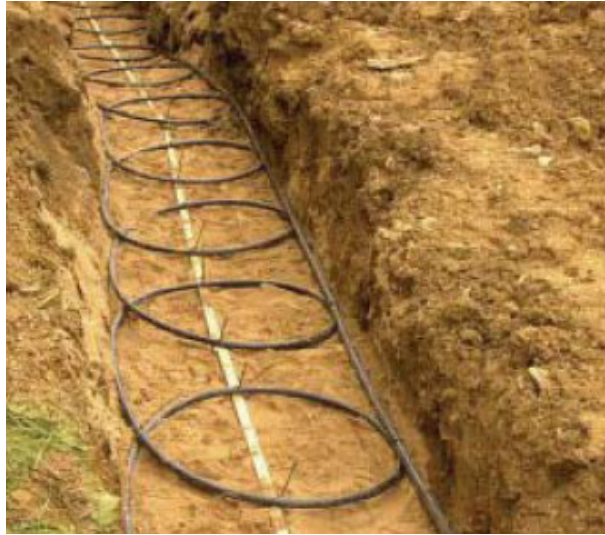
Figure 7.5.7 – Installing Spiral Coil (LCBP, 2004)
