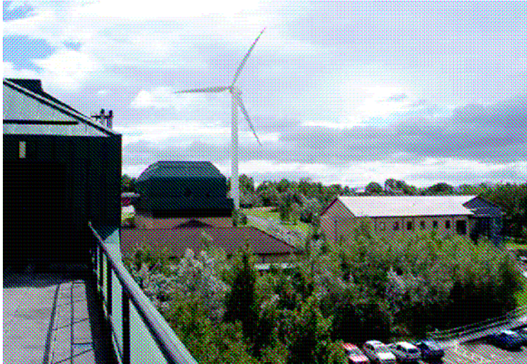
Figure 9: 660kW wind turbine installed in Antrim Area Hospital (71)
