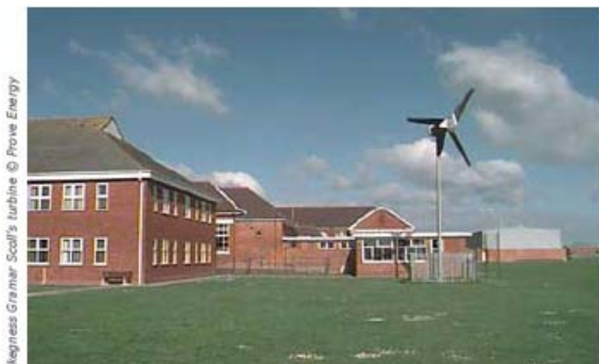
Figure 4: Wind Turbine Installed in a High School Premises (4)
