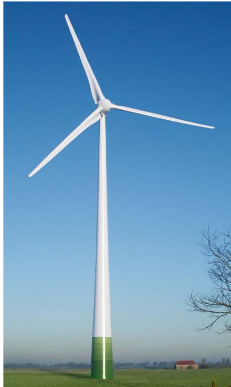
Figure 18: The ENERCON E-82 wind turbine
