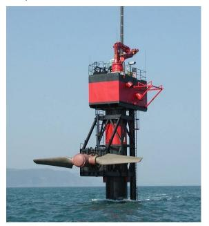
This is the type of device upon which the channel model will be based. The turbine could conceivably have either a single rotor as shown in figure 7 or a twin rotor configuration as is shown in figure 8. The rated power of the former is approximately 500kW and the latter a full 1 MW.
