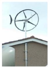
manufactured by Renewable Devices based in Edinburgh, Scotland. The turbines can be utilised for grid – connected embedded power generation, installed with a battery bank for off-grid stand – alone applications or linked to an immersion water heating system.
