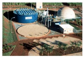
figure 5. A digester treating dilute wastewater at a fuel ethanol production plant in Brazil
