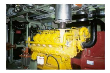
figure 9.Biogas use in internal combustion engine
