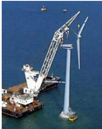
Figure 5: Installation of a 500KW Vestas wind turbine at Tunoe Knob-Denmark
