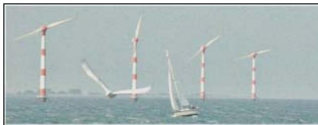
Figure 6: The four 500kW Nedwind wind turbines of Lely's wind park
