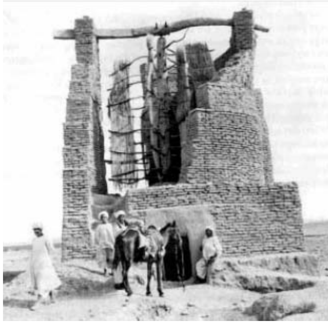
Figure 1: The oldest construction used for the production of energy from wind
