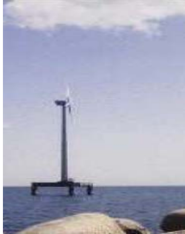
Figure 3: The first offshore wind turbine at Nordersund-Sweden
