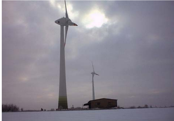
Figure 55: Enercon E-112 wind turbine
