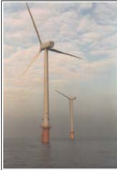
Figure 7: The two Vestas wind turbines of Blyth's wind park
