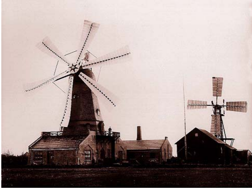
Figure 2: The first wind turbine at Askov
