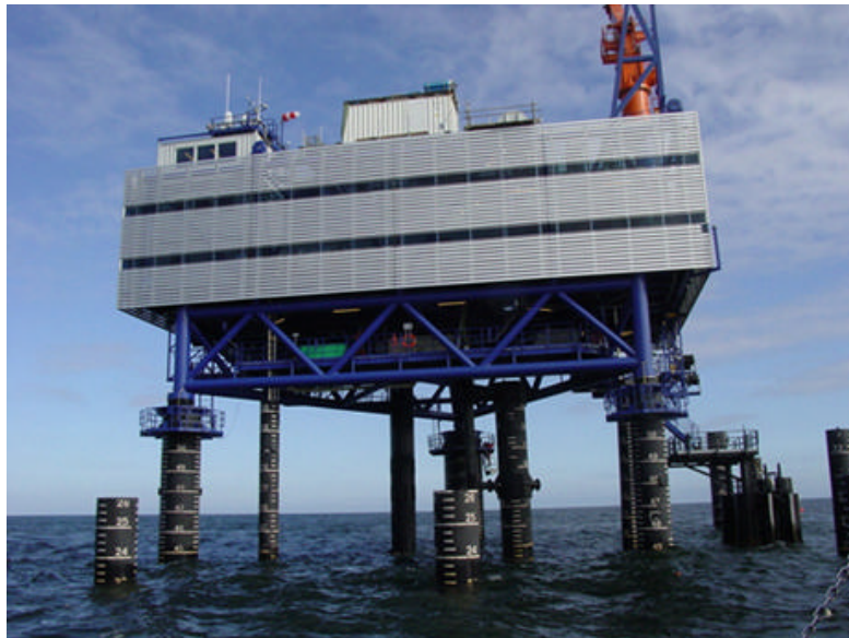
Figure 2.9 A photo of the transformer substation module at Horns Rev OWF [14]
