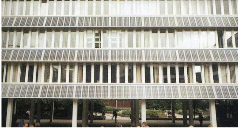
Figure 4.2 Britain's first building with PV cladding, a 40kWp system installed in 1995 on the façade of a refurbished computer centre at the University of Northumbria, Newcastle
