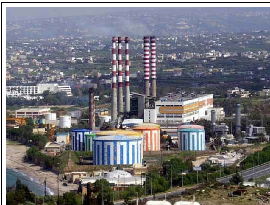
The Power Plant in Linoperamata
