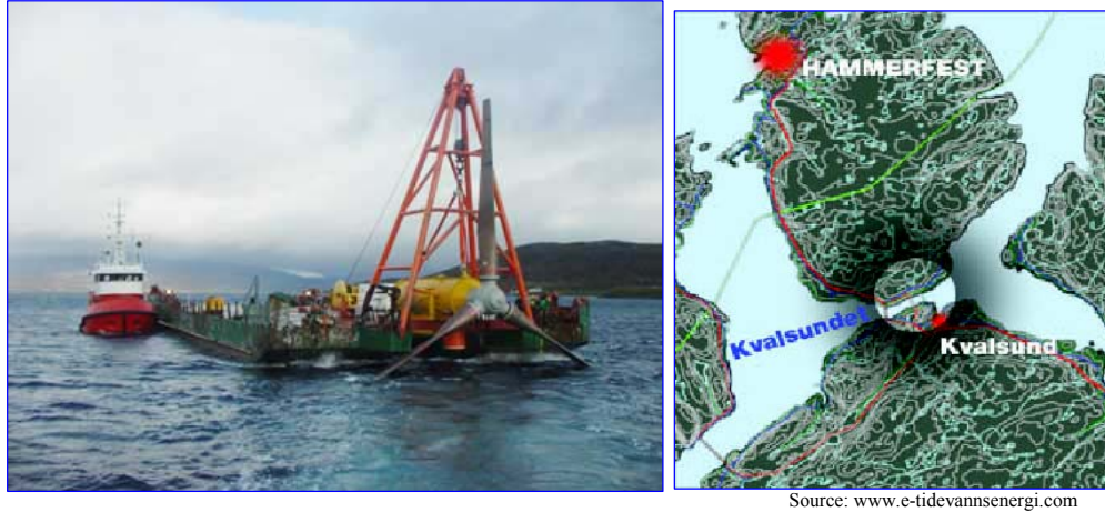
Figure 2.6 Deployment of the first grid connected tidal turbine in Kval Sound, Norway
