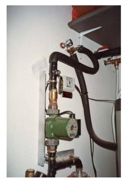
Figure 5.6.8.2.1: Temperature control system. The small screen shows 84 °C.
